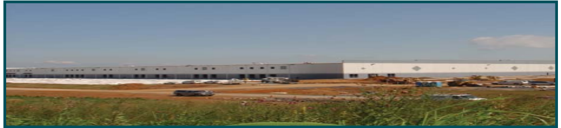
Kellogg's will occupy 215,460 sf of the newly constructed 554,000 sf facility
